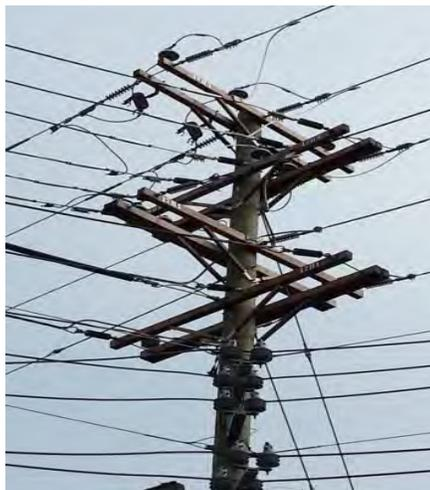
Eversource completed a Distribution System Study for the 4.16kV system in downtown Nashua in March 2016. This study supports the rebuild of the Millyard SS with two (2) 34.5-4.16kV transformers and six (6) feeder circuits. The study recommended two (2) 5MVA transformers but the design criteria has since been updated so two (2) 10 MVA transformers are now
